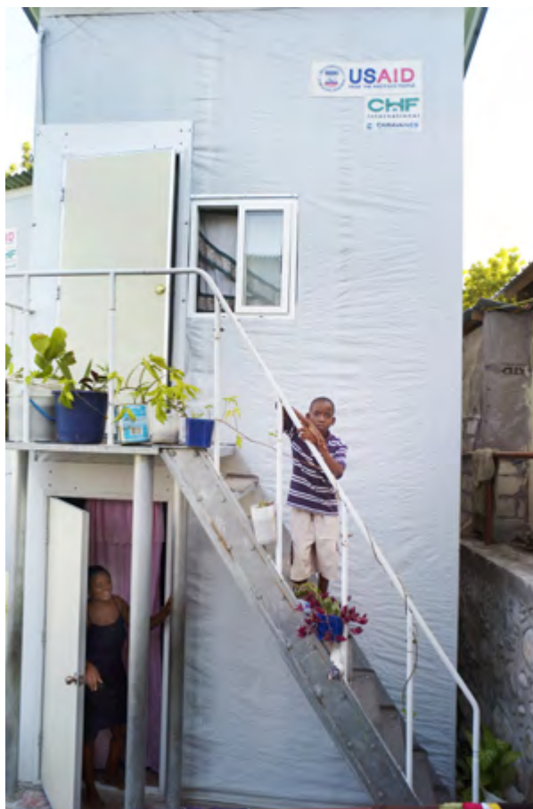
Residents in new housing in Ravine Pintade, a hilly area in the center of Port-au-Prince which was previously damaged by the earthquake. An extra floor was added to address the small size of the plots. Photo: CHF/Maggie Steber, May 2012
