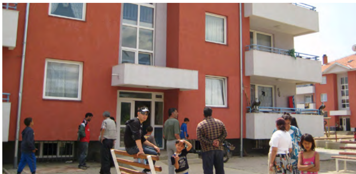
View of the destruction of Roma Mahala after the conflict, and of a rehabilitated building. Photo: IDMC/B. McCallin, May 2009
