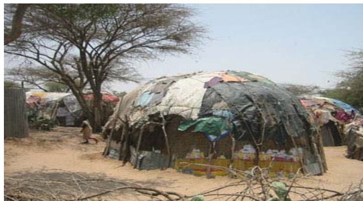
Typical IDP huts made out of old rags, plastic, ropes and sticks, Hargeisa, Somaliland. (Eschenbacher/2004)
