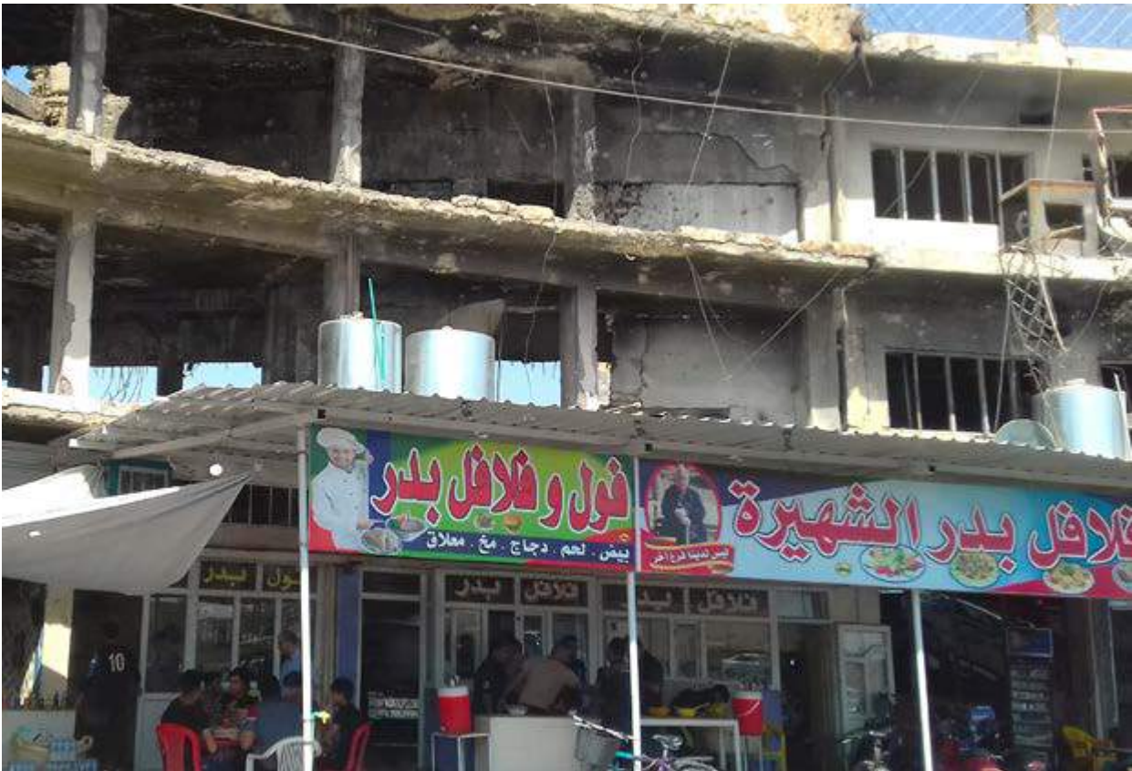
A restaurant in a damaged building in west Mosul
