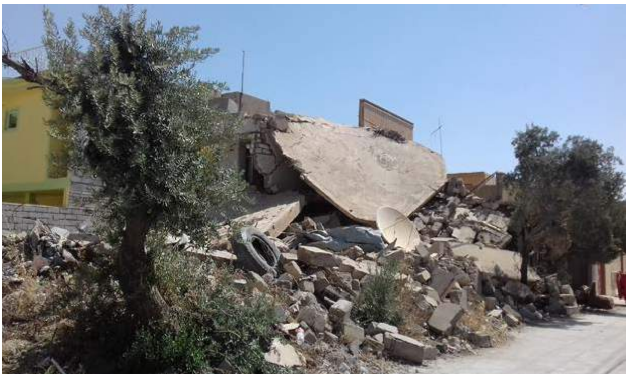
A destroyed home in Bashiqa
