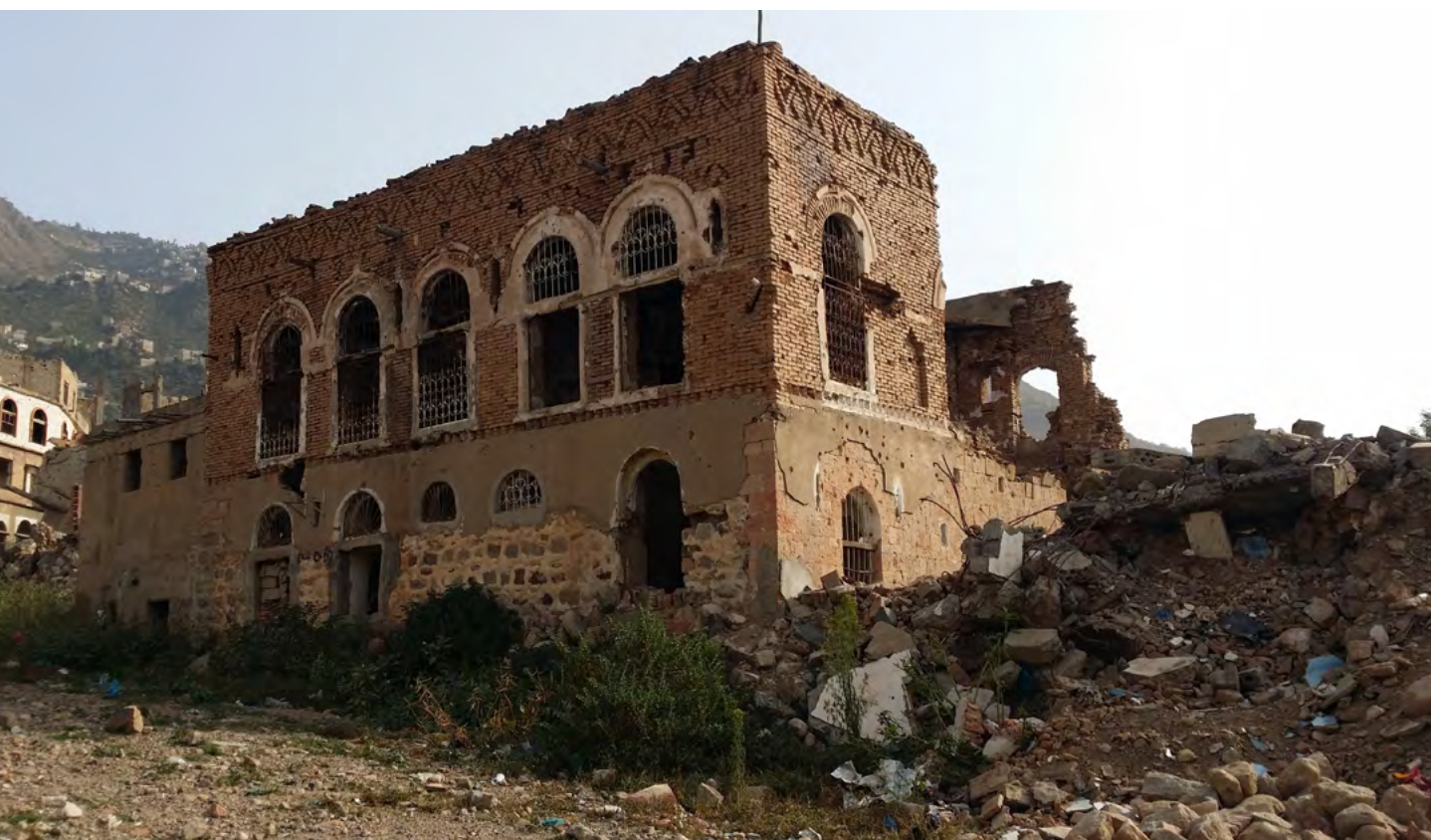
Destroyed buildings in Taiz city, Yemen. Photo: Akram Al-Sharjabi, August 2019
