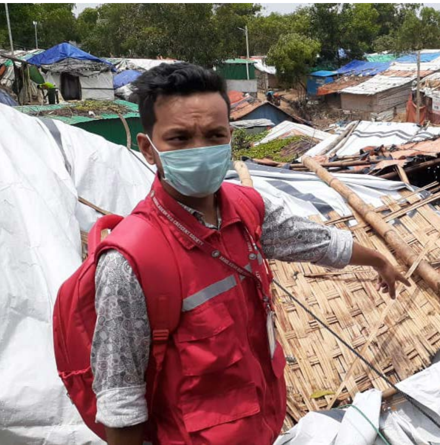
Destruction after Cyclone Amphan in Cox's Bazar, Bangladesh, May 2020. © BDRCS
