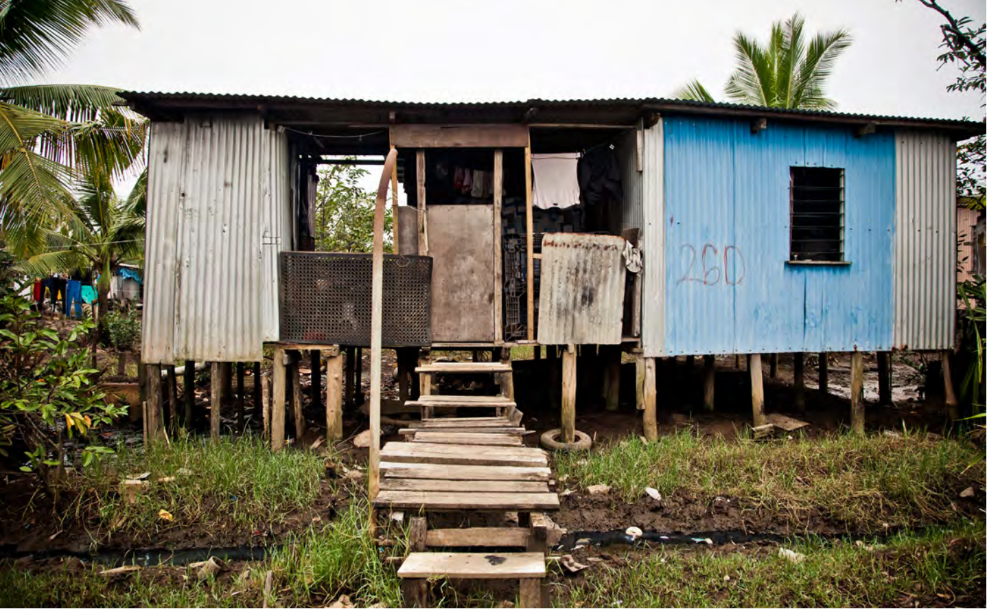
Floods are very frequent in Waelea settlement, Suva, but the biggest issue is the lack of sanitation. All the houses have toilets which flow directly on the ground carried by a constant stream of dirty water. © Benoit Matsha-Carpentier/IFRC, Fiji, May 2013.
